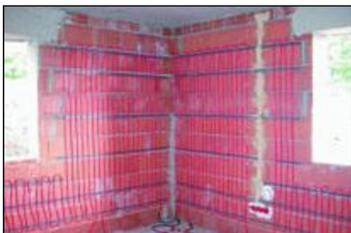
Figure 11: Wall heating/cooling system.
