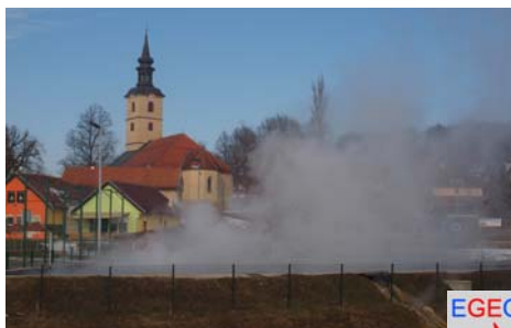
Geothermal well in Benedikt, Slovenia
