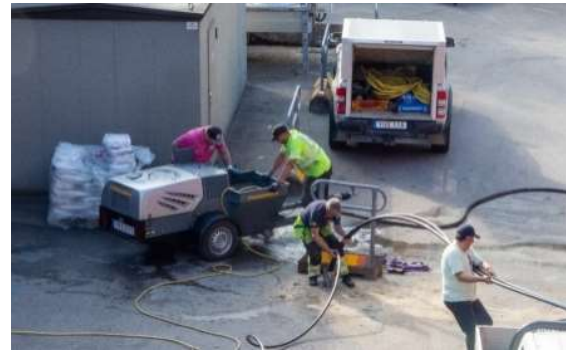
Figure 16: Grout mixing and injection at RISE Borås.
