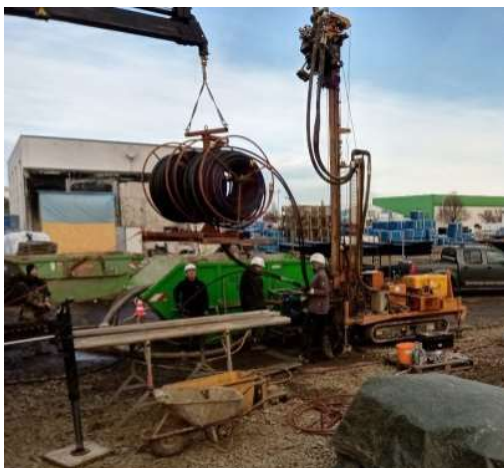
Figure 11: Insertion of GEOCOND double-U pipe from reel lifted above borehole.
