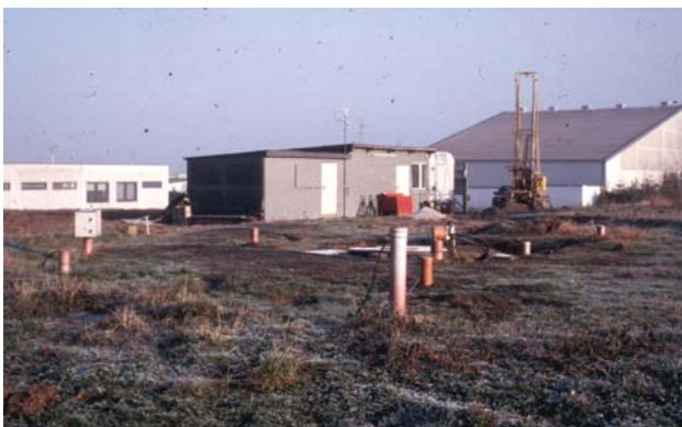
Figure 10: Schwalbach GSHP-research station on a very cold day in January 1988
