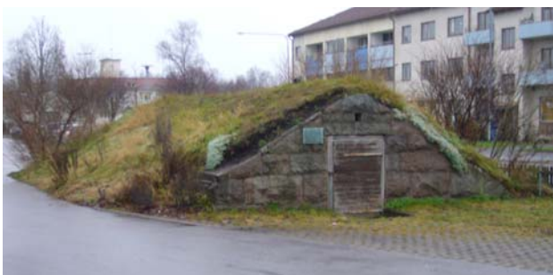
Figure 1: Storage shed partly underground in Emmaboda, Sweden, amid modern houses in 2007
