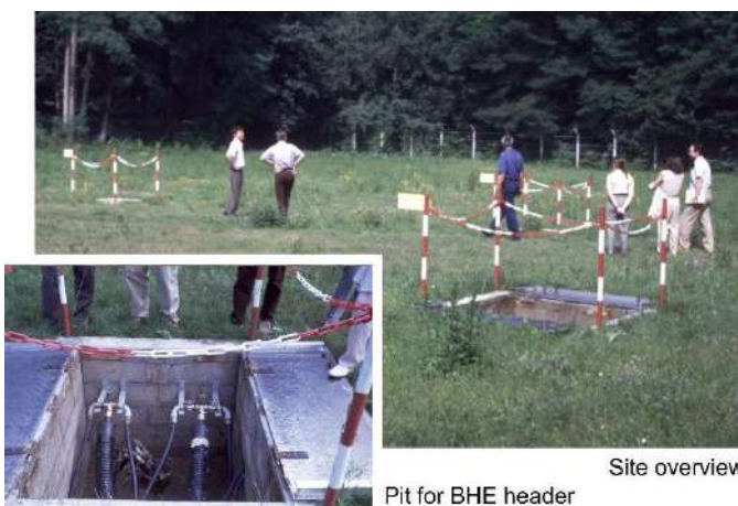
Figure 12: BHE test site at EdF laboratory les Renardières near Moret-Loing-et-Orvanne, France, July 1999.
