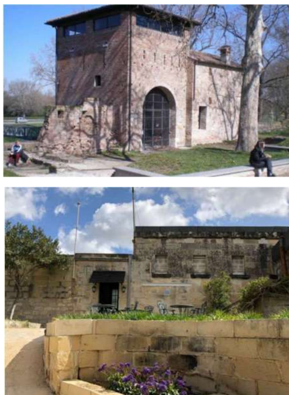
Figure 34: Two examples of historic buildings equipped with GSHP using BHE; above Porta degli Angeli, Ferrara, Italy, below Msida Bastion Historic Garden, Valletta, Malta (from GEO4CIVHIC project).
