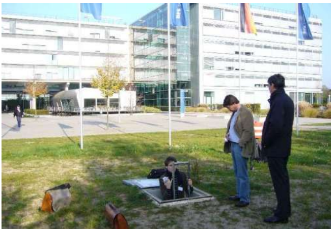
Figure 19: Headquarters of DFS in Langen, Germany, seen from the site of the BHE field; the manhole in the foreground gives access to one of the large manifolds (photo from October 2007).
