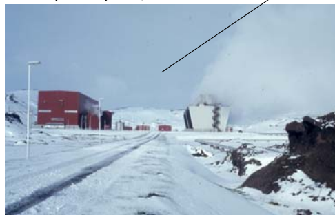
Krafla power plant, Iceland
